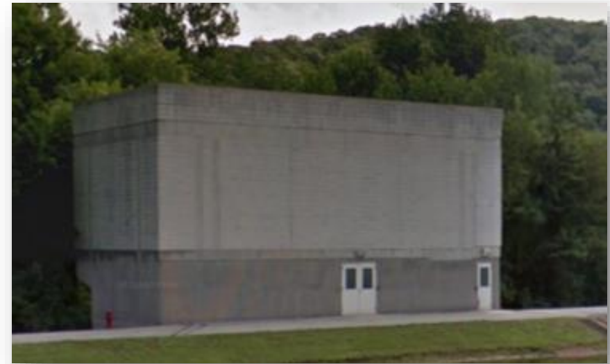
Raw Water Pump Station (built 1992)
